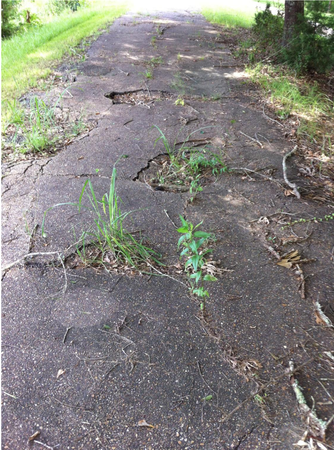
Photograph 5. Close up of broken asphalt and pot holes on top of dam.
