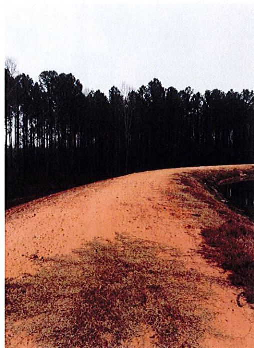
Looking South from Station 4+00; Dam Crest on south end; recently rehabilitated; Vegetation Required
