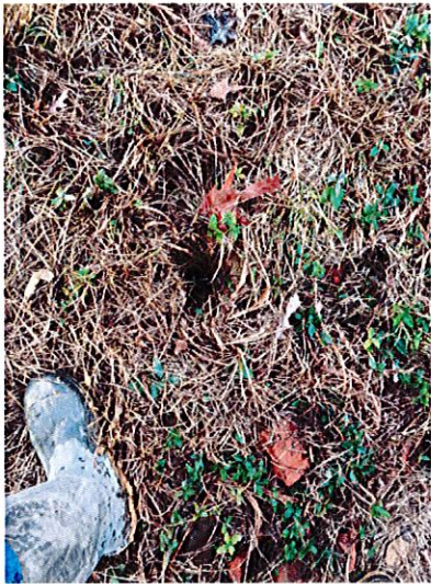
Multiple rodent burrows/holes on upstream slope all along the levee
