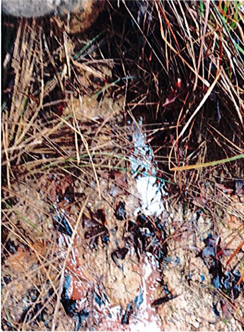
Seepage in stream beyond downstream slope – Right of Station 3+00. Iron bacteria results in orange water and oily sheen.
