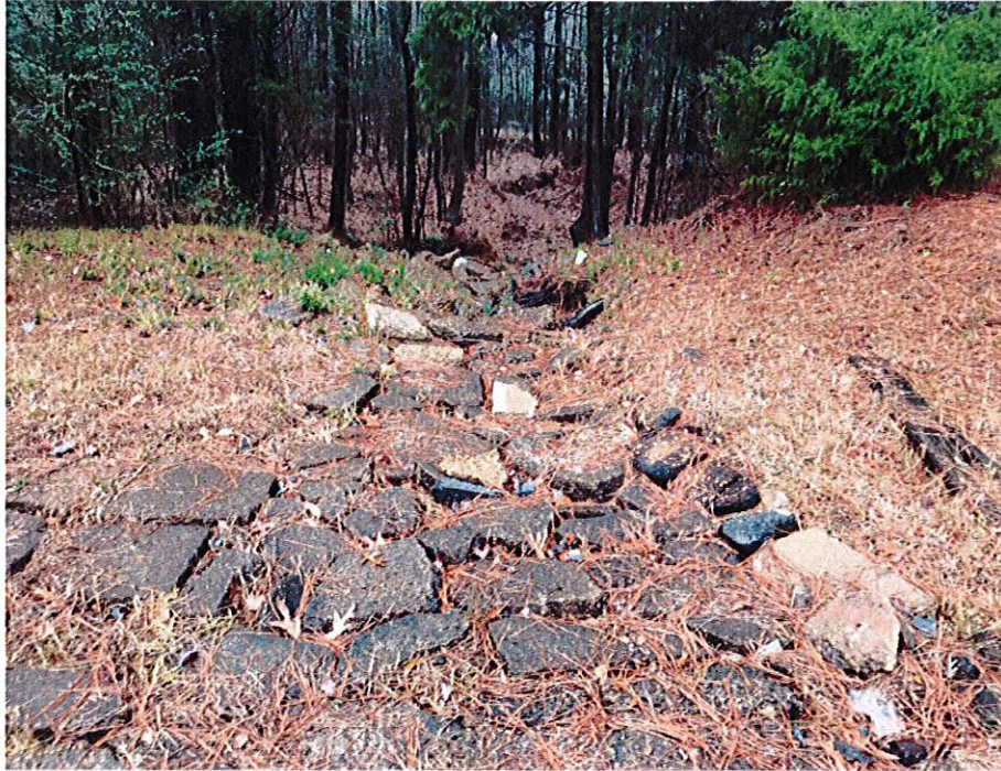
Primary Spillway - concrete rubble exit chute
