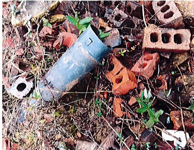
Black steel pipe protruding out of upstream slope – Station 9+00; unknown purpose
