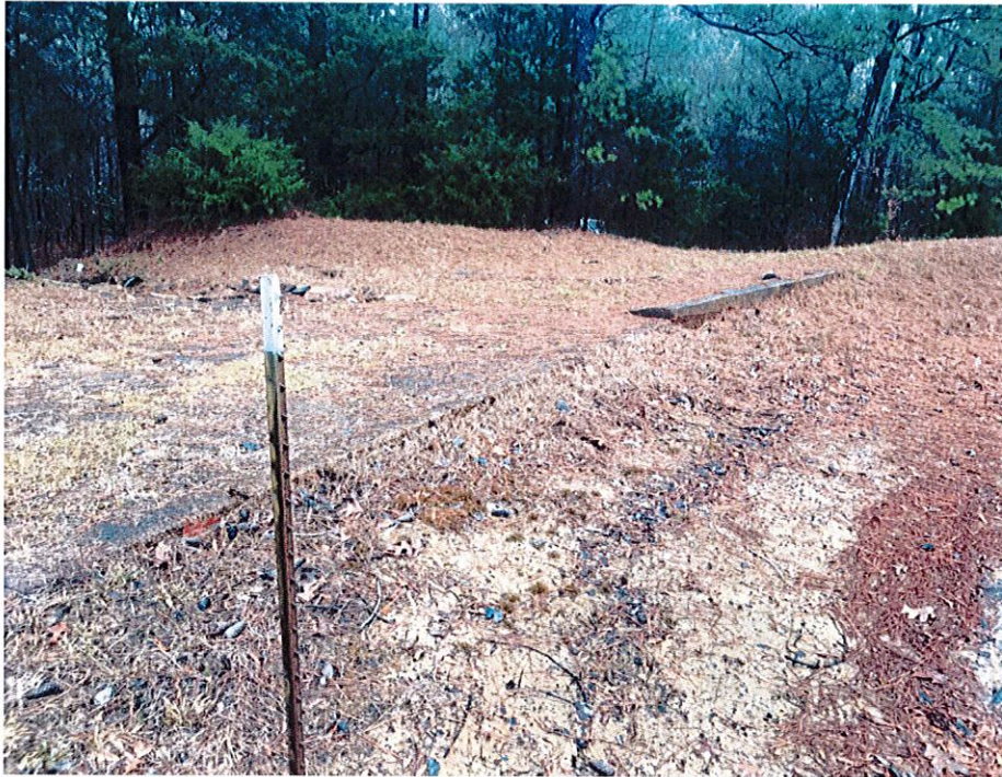
Primary Spillway - weir and concrete control section
