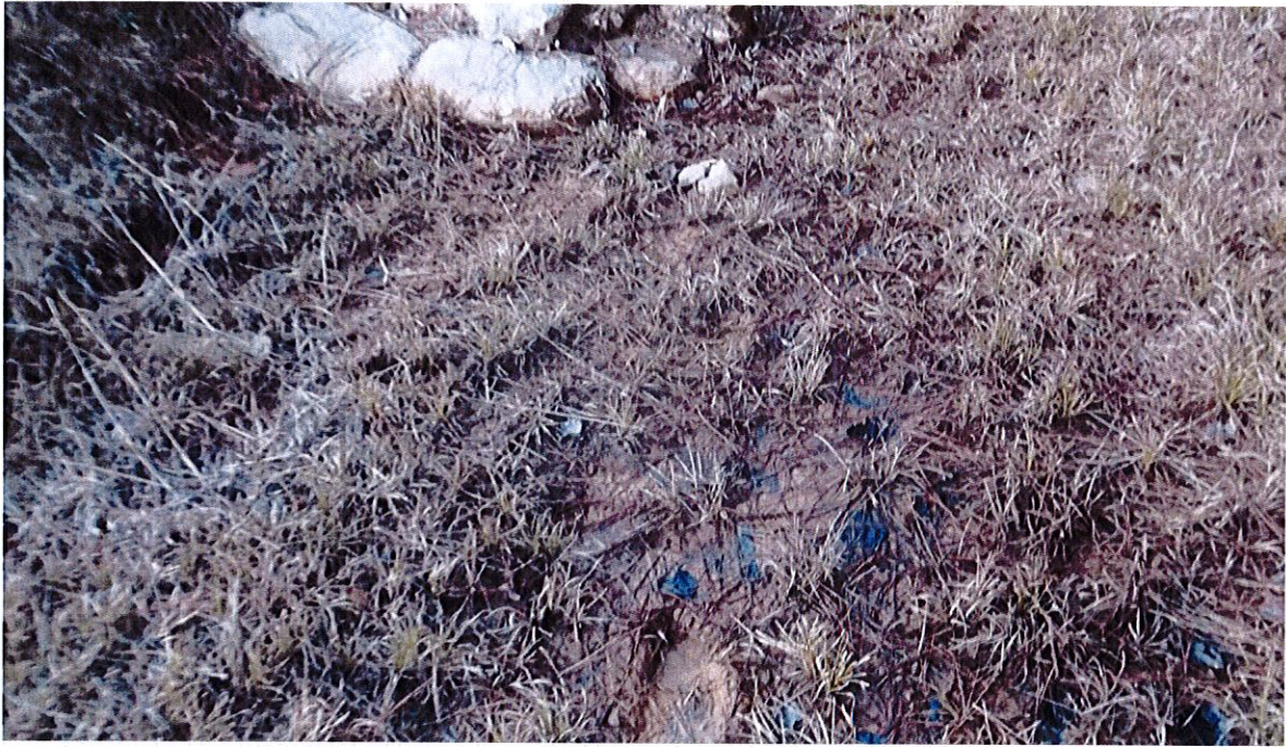
Downstream Slope Right of Station 9+00 - Seepage on the lower bench next to sandbagged area
