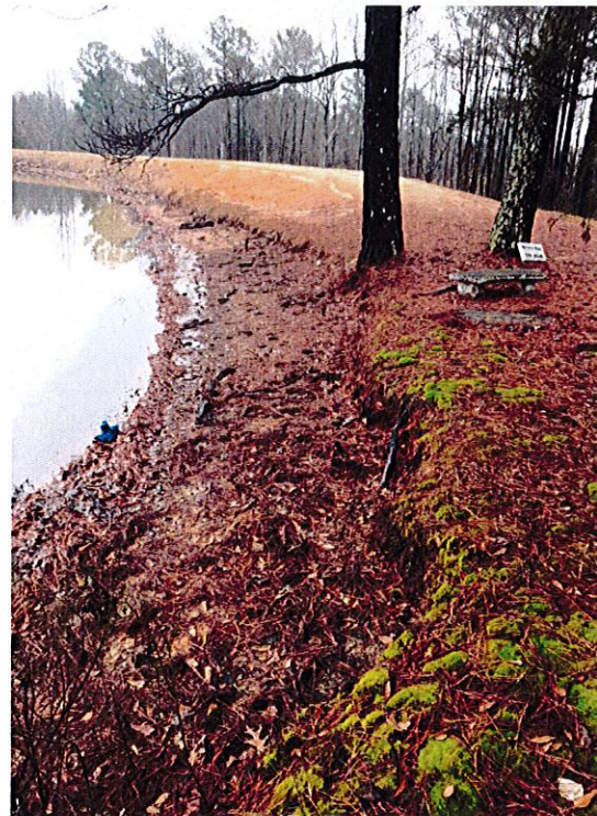
Scarp - wave action eroding bank at Emergency Spillway
