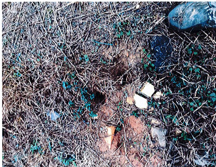
Multiple rodent burrows/holes on upstream slope all along the levee
