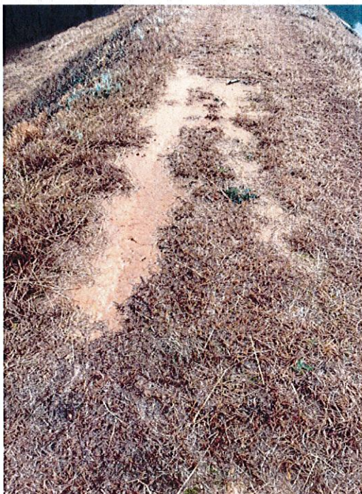
Vegetation wearing on dam crest; Station 6+50
