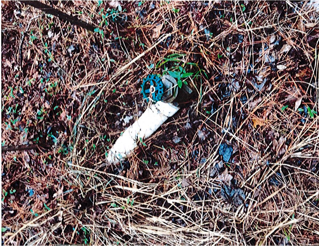
Level Control Piping Valve - 4" PVC pipe with brass valve – At downstream slope toe right of Station 6+15.
