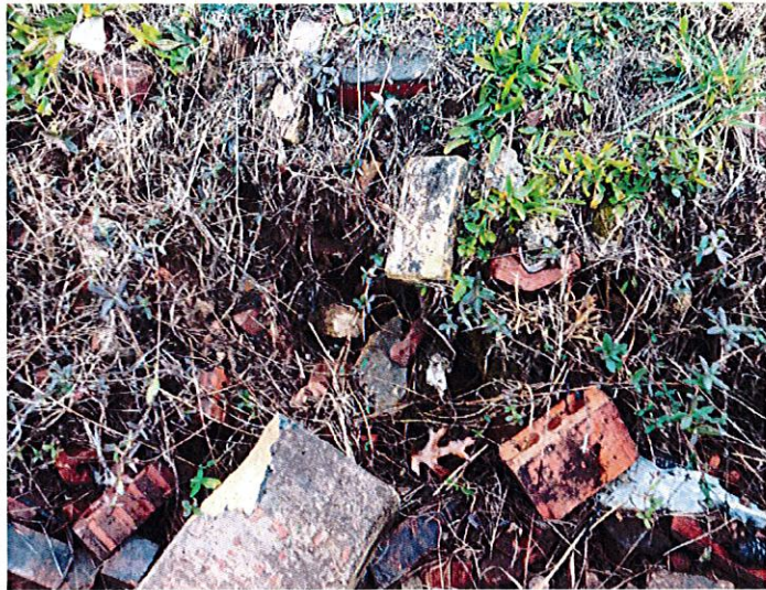
Multiple rodent burrows/holes on upstream slope all along the levee
