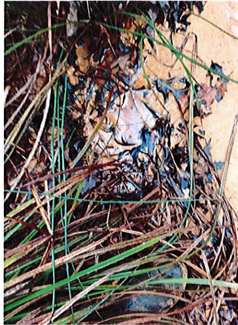
Seepage in stream beyond downstream slope – Right of Station 3+00. Iron bacteria results in orange water and oily sheen.
