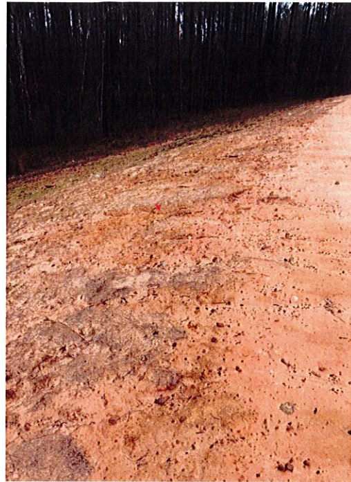
Rill and gully erosion forming on crest and upstream/downstream slopes at south end of levee
