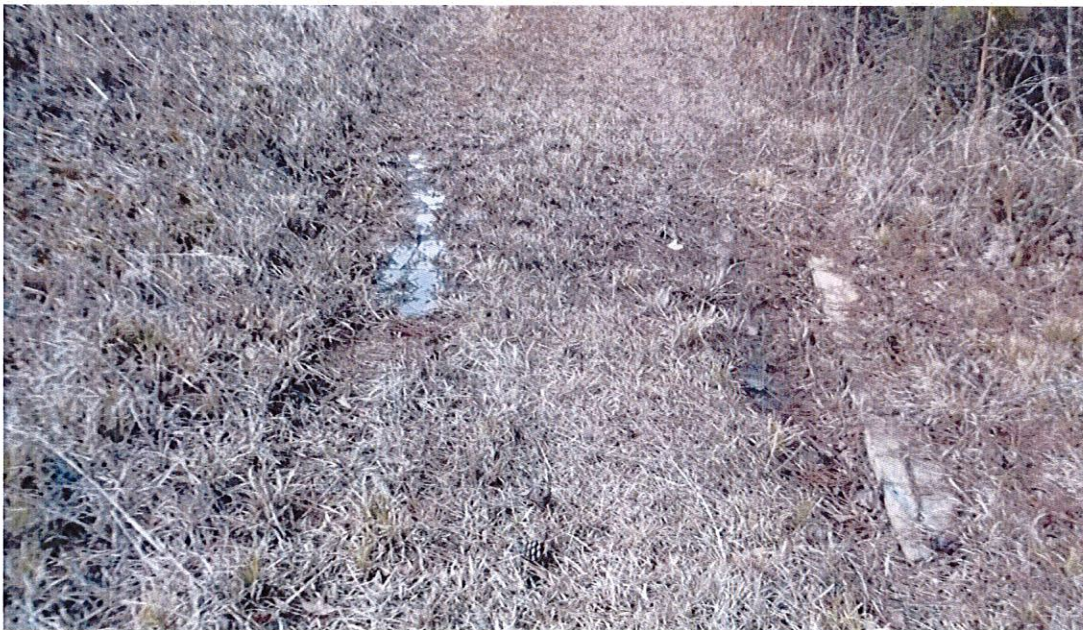
Downstream Slope Right of Station 8+50 - Seepage on the lower bench
