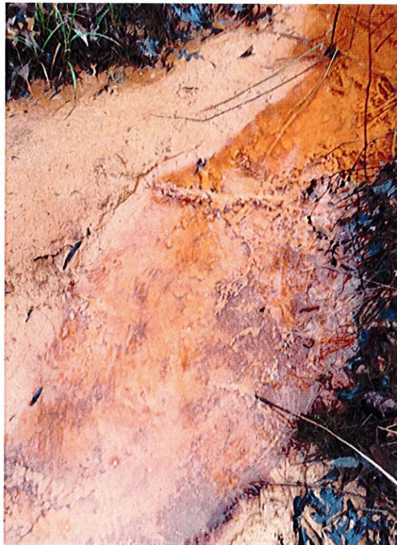
Seepage / flow in stream beyond downstream slope right of Station 2+00
