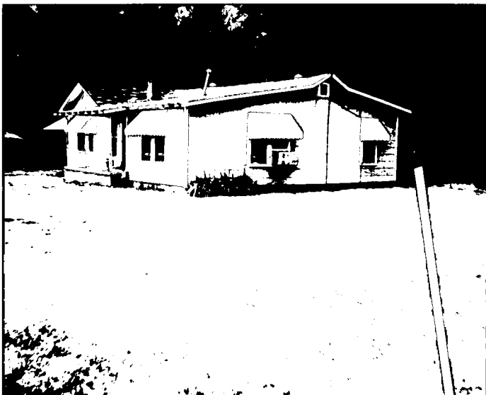
Well house in back M3 Union
